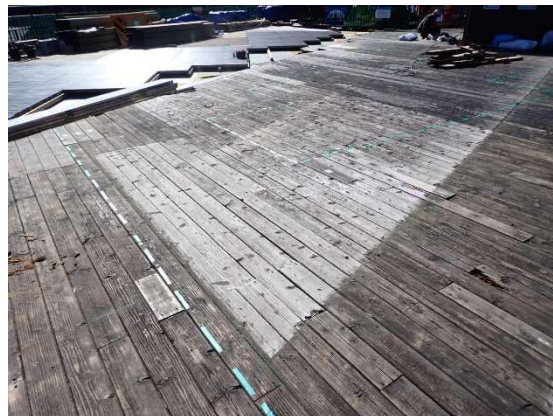
(山麓修繕実施箇所)
